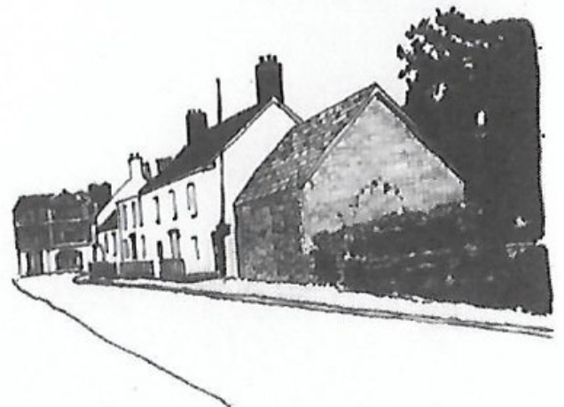
27. Site of Porthycarne Gate Porthycarne Street (W)
